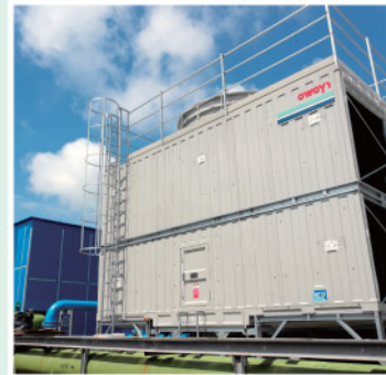
▲ Replacement of air-cooled chillers with energy-efficient water-cooled chillers
