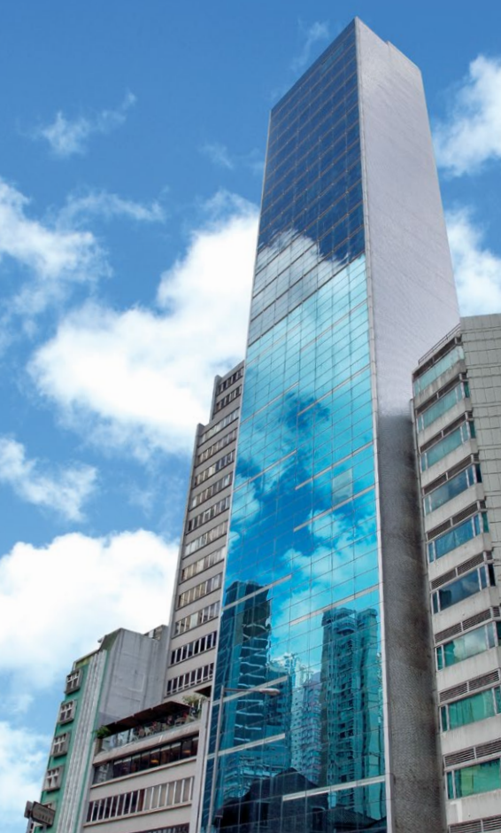
Winsome House Property
