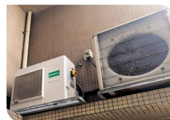
Replaced with new split-type air-conditioning unit
